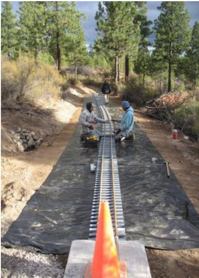
Right - Gil Domingez delivers track panels to Hope Circle Left - Dustin Barnes and Paul Aragon connect the last track panel south of the Panzik Road Crossing. Chris Curtis walks down the track to start cleaning up the tools.
